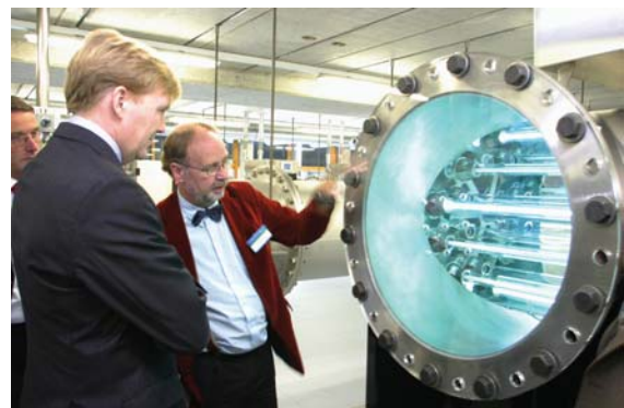
UV for disinfection at Andijk (PWN 2005)
