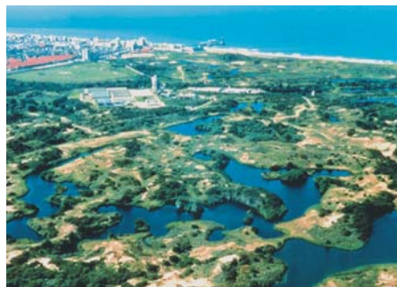
Infiltration ponds in the dunes along the North Sea coast at The Hague
