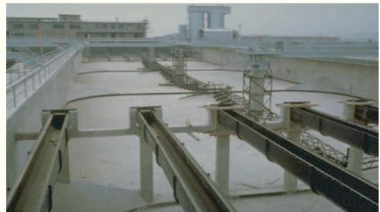
Figure 24 - Outlet construction: overflow weir for effluent discharge
