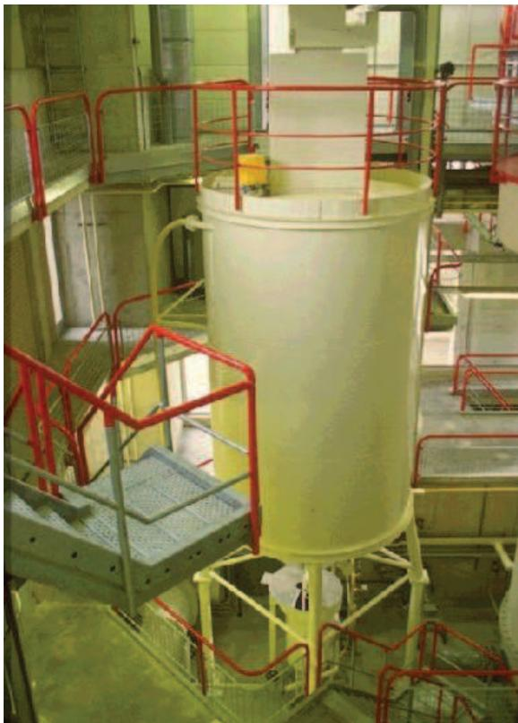
*Figure 10 - Seeding sand storage silo with sand washer underneath*
