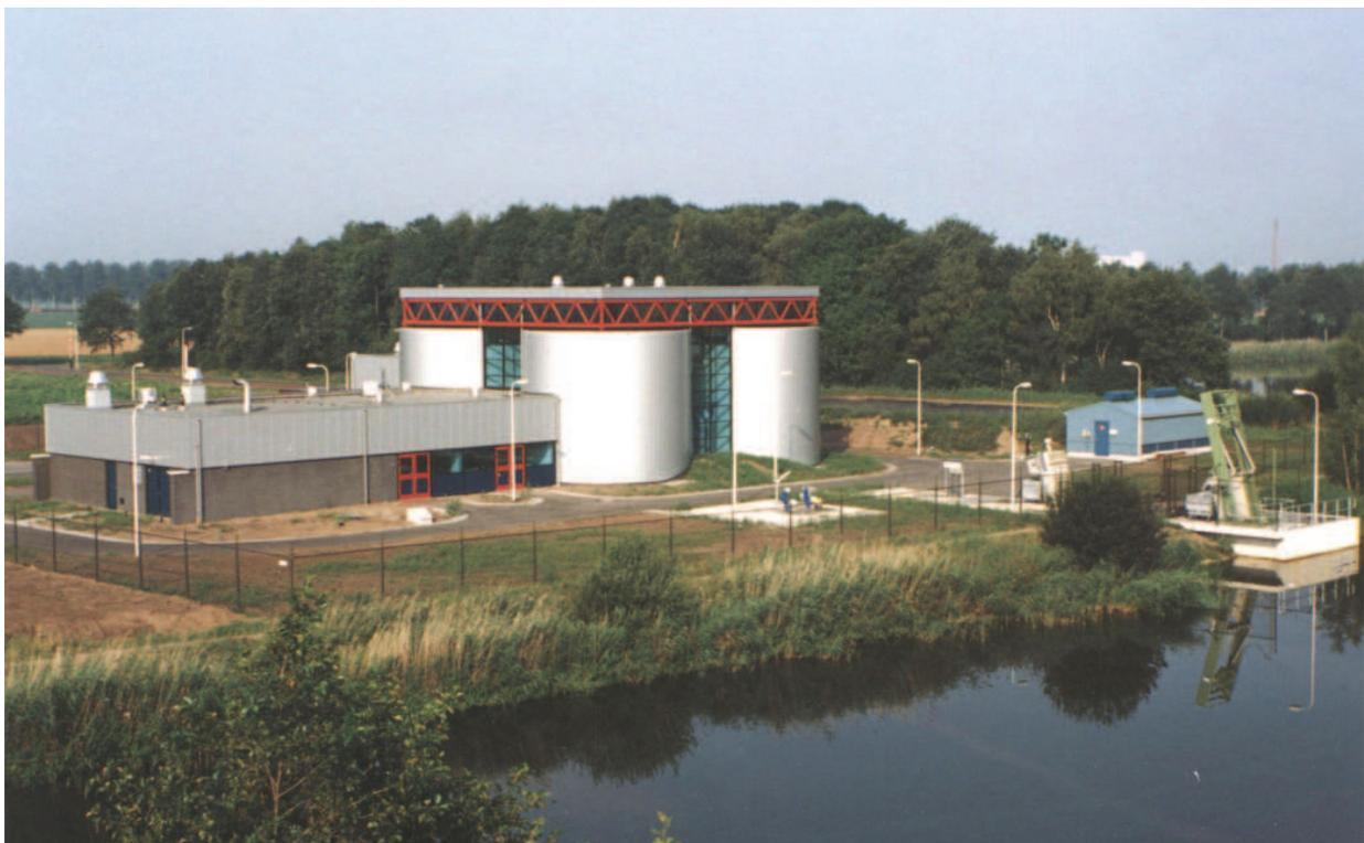
Figure 9 - Industrial water project Veendam (Groningen) with anaerobic injection water from surface water
