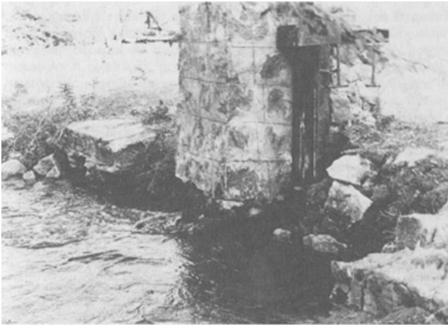
Photograph 4 Half demolished stone-and-mortar pipe outlet with gate frame still visible
