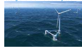
Floating wind farm [9]
