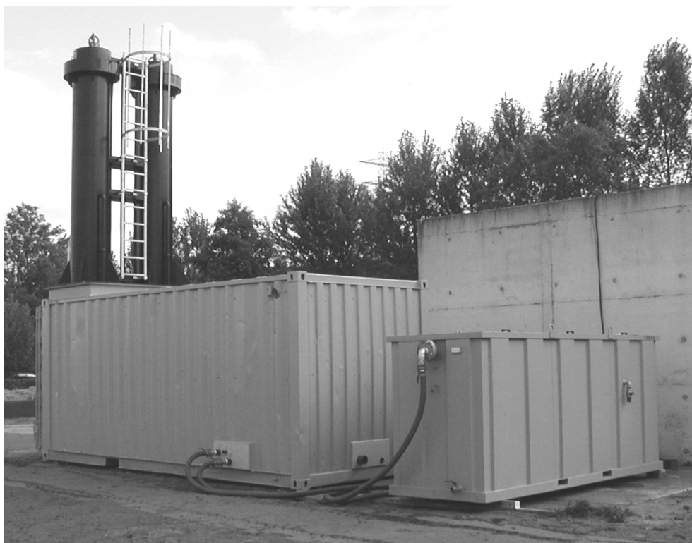
Figure 5 The two reactors of the pilot plant at WWTP Ede, with other equipment in the container and the tank to pre-settle incoming sewage
