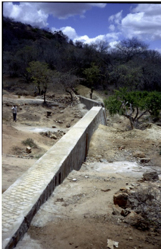
Figure 3. Almost completed dam in the dry season
