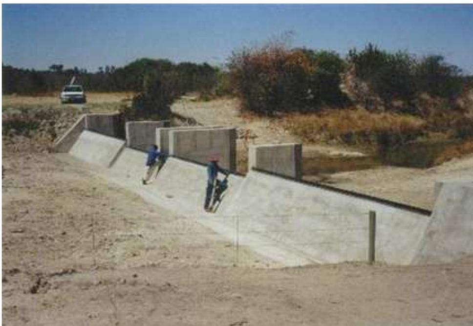
*Fig. 8.41: Compound gauging weir under construction (Zimbabwe, Mupfure catchment)*
