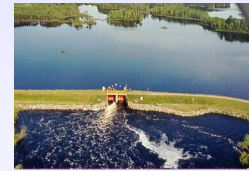
Spirit reservoir dam near Wisconsin river
