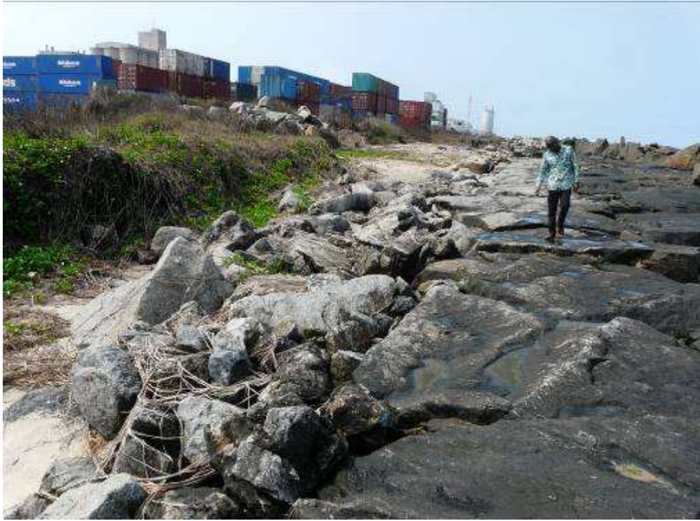
9) View of the container stockyard from the existing breakwater
