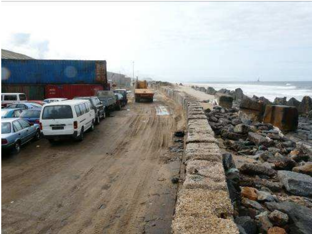
6) Access road to existing breakwater
