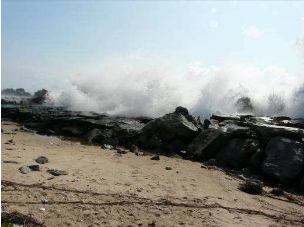
11) Wave overtopping on existing breakwater in normal conditions
