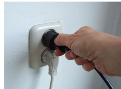
Ready to go, plugging it in.
