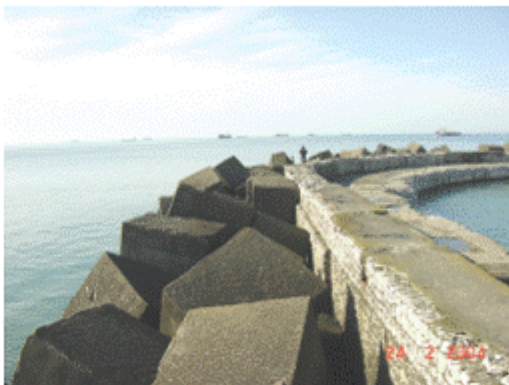
Figure 4 Breakwater chainage 0-1040 m
