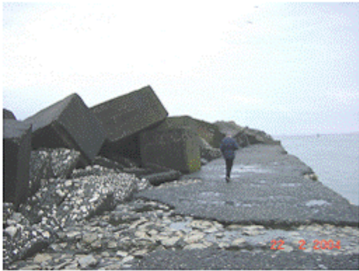
Figure 6 Breakwater chainage 1040-1270 m
