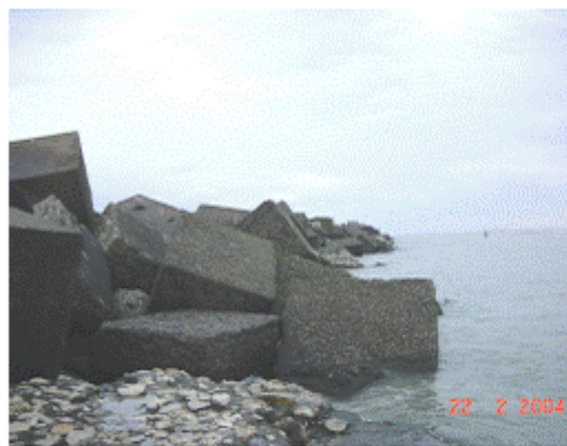
Figure 8 Breakwater chainage 1270-1810 m
