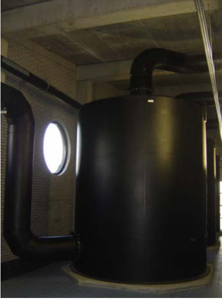
Figure 2.3: In this picture is represented one of the tower aerations present in the plant of Harderbroek. It is located in a room above the filters and it is receiving the water by means of a pump.
