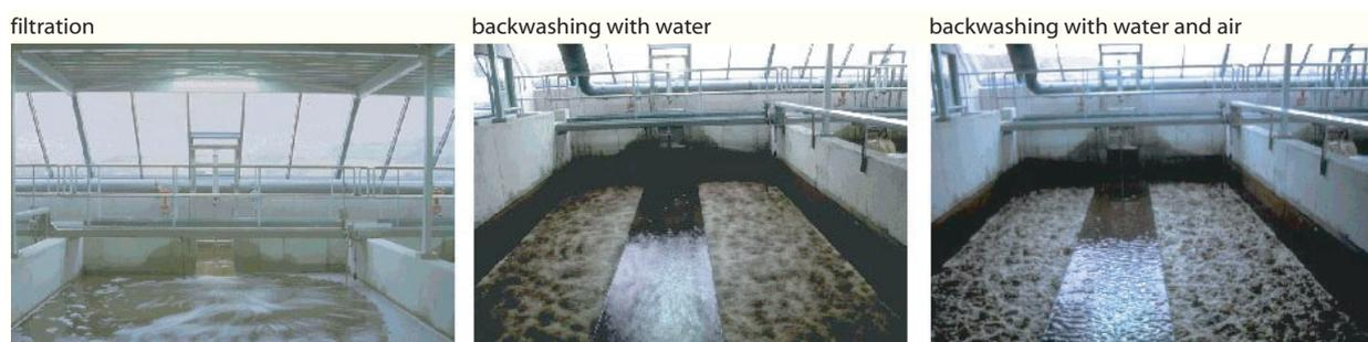
Figure 8 - Filtration, backwashing with water and air
