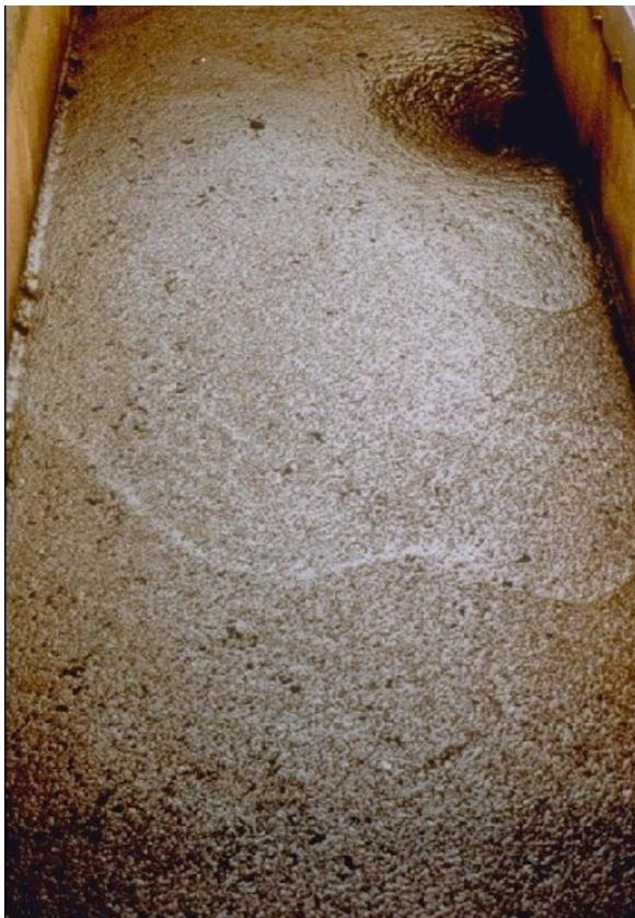
Figure 20 - Result of a poorly designed filter bottom
