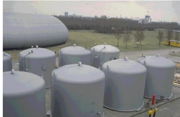
Figure 26 - Cylindrical steel pressure filters
