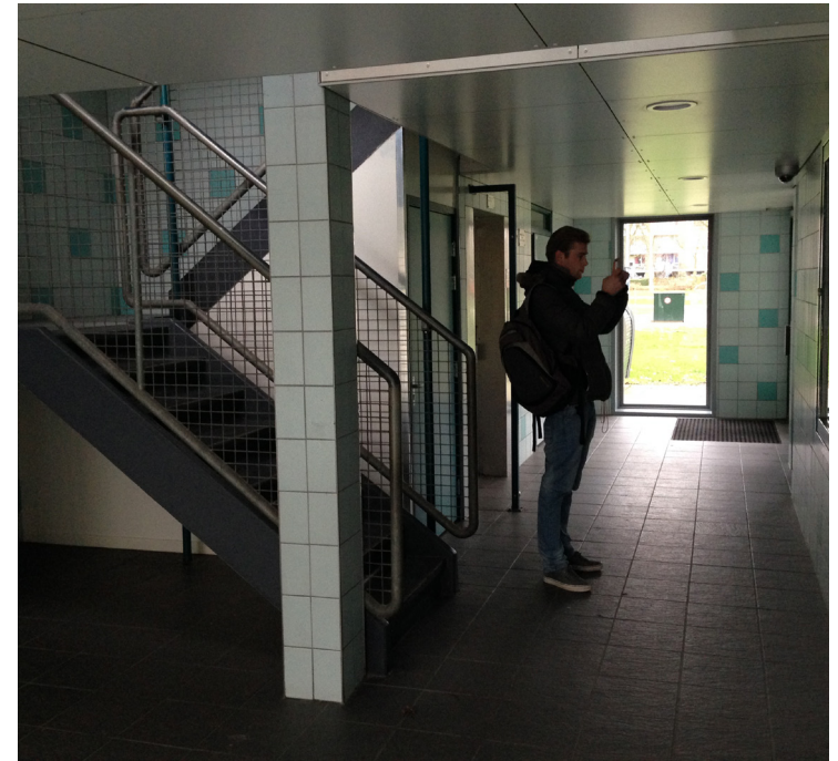
FIGURE 1.4.3. STAIRCASE AND LIFT AREA
