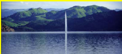
A permanent fountain discharges the CO 2 inflow in Lake Nyos (Cameroon) to prevent the recurring of the 1986 disaster [16] .
