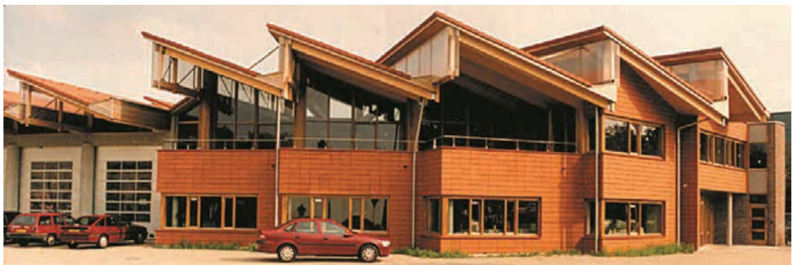
Fig. 04.77: Backside of the fire-station in Soest.
