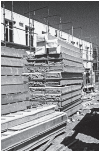
Fig. 04.06: The piled-up rafter roof elements with thermal insulation (left) and the roof with integrated Velux windows just before the roof tiling works
