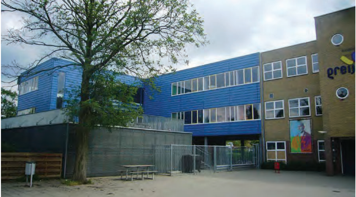
Fig. 04.81: Front of the Greijdanus School, the new build left to the original building,
