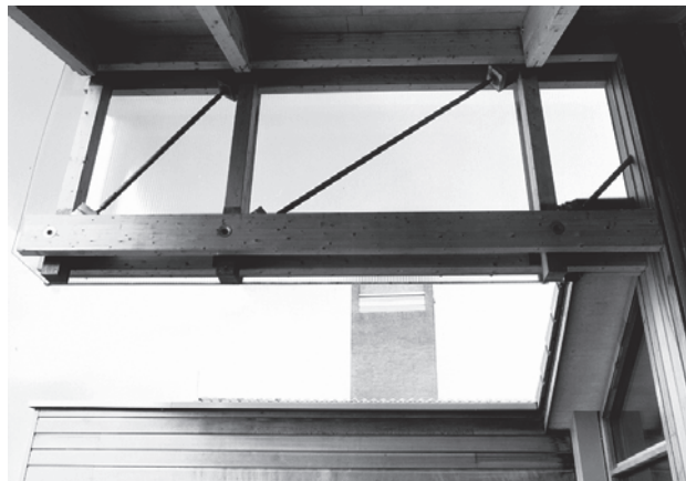
Fig. 04.79: Hammer-beam truss, covered with transparent polycarbonate plates and with the old firehose tower on the background.
