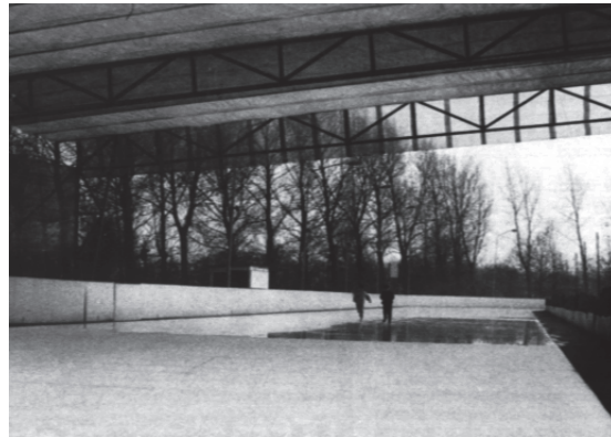
Fig. 04.49: Free-cooling test roof in Haarlem 15
