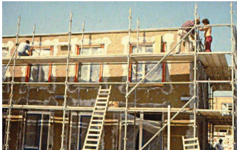
Fig. 04.03: The plasterers are working outside one of our well-insulated houses in the 1980s. Extra reinforcement was applied in fragile places at the edges of the window-frames. One had no experience, so everything was done as safe as possible.
