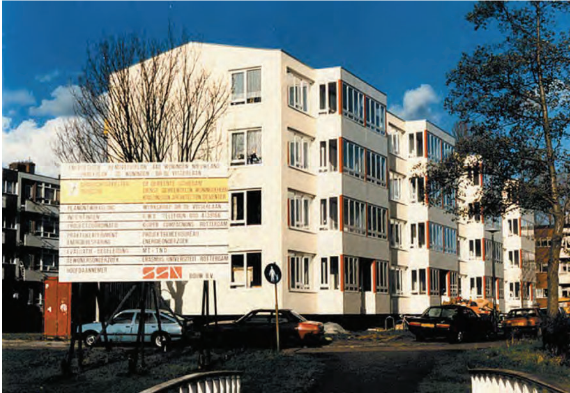
Fig. 04.18: Font side of the tenement flats in Schiedam after renovation
