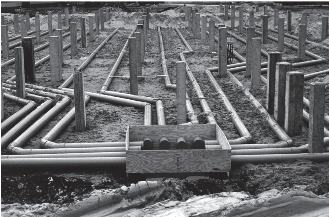
Fig. 04.65: Piping required to harness soil energy
