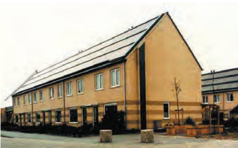
Fig. 04.86: Dwellings with solar collectors (left) feeding the inter-seasonal heat storage (right) for 100 dwellings in Beijum.
