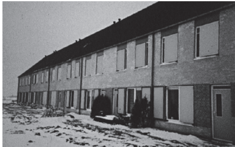
Fig. 04.10: Test of thermally insulating shutters in the Beijum district of Groningen (left) and the ones applied in the neighbourhood of Woudhoek-Zuid in Schiedam (right)
