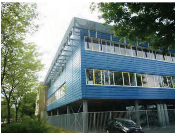
Fig. 04.82: Mesh foot-racks act as sunshading device at the roof cornice.
