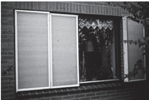
Fig. 04:15: Translucent insulating shutters seen from the outside and inside
