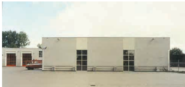
Fig. 04.71: Garage (left) and north-west elevation (right). The air-pipes lay under the fire engine garage, which has a roof of steel Litzka beams. Grates for air inlet can be easily distinguished in the facade.
