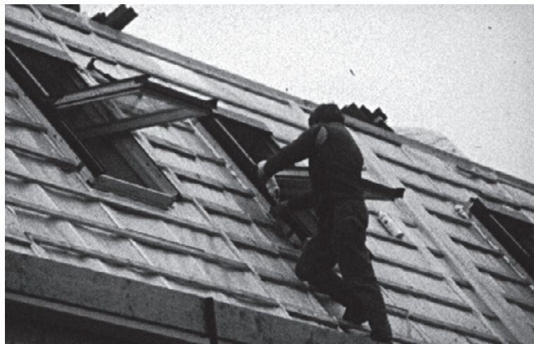
Fig. 04.06: The piled-up rafter roof elements with thermal insulation (left) and the roof with integrated Velux windows just before the roof tiling works
