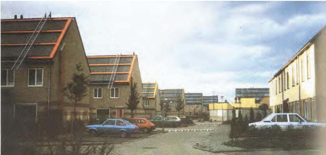
Fig. 04.85: Installation of solar panels to be combined with an inter-seasonal store, extension Beijum, Groningen, 1982.
