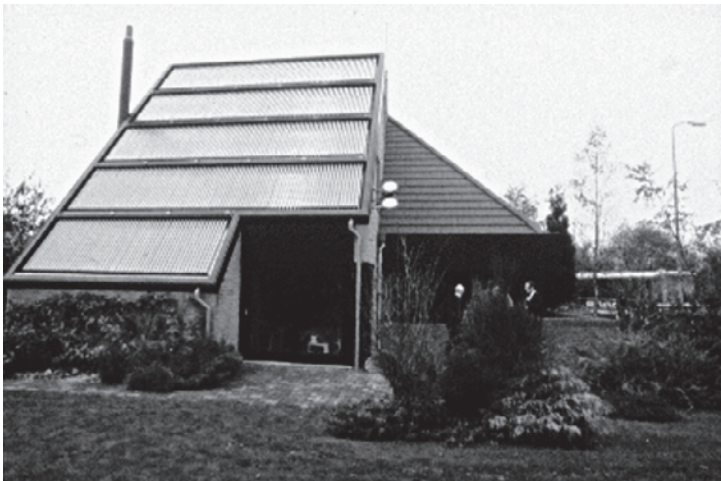
Fig. 04.88: Solar panels in-situ at the Prof. Van Koppen residence (Architect: A. Hoekstra), Eindhoven, 1981 (left), with high-tech vacuum collectors and warm water storage tank of 3.7 m 3 . Detail of the vacuum tube heat pipe collector (right).
