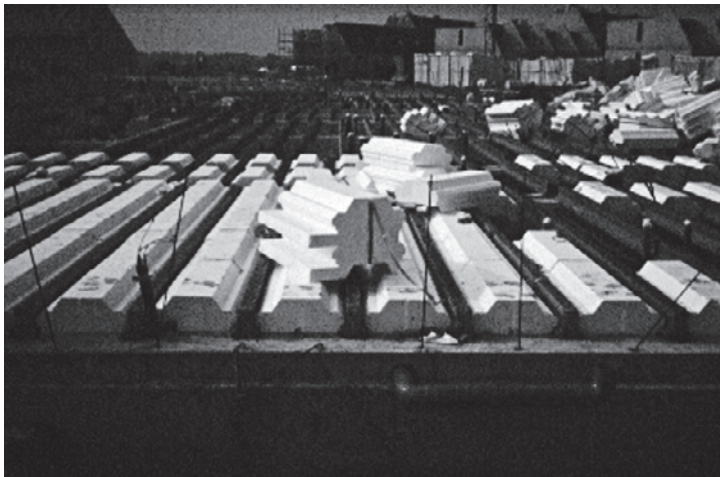
Fig. 04.02: Polystyrene cushions placed between pre-stressed concrete beams
