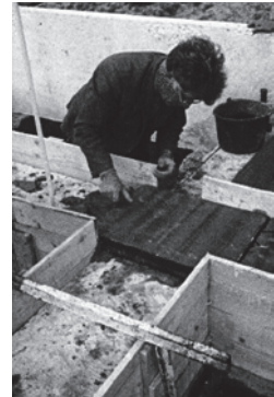
Fig. 05.30: Placement of heavy load-bearing foam glass in the foundation.
