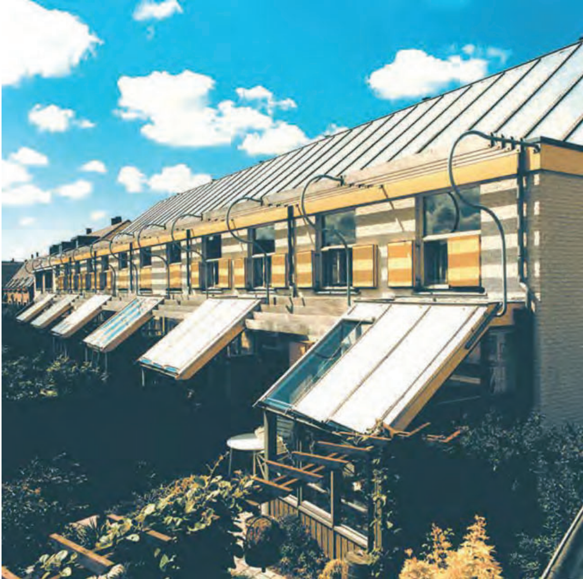
Fig. 05.28: The nine Solar Cavity Wall Dwellings with fixed wooden sunshading on the first floor and external sunshading on the conservatory roofs to avoid overheating.
