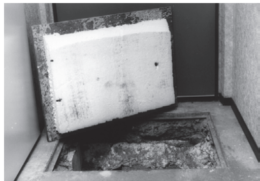
Fig. 05.19: Insulated panel to the crawling space behind the front door.
