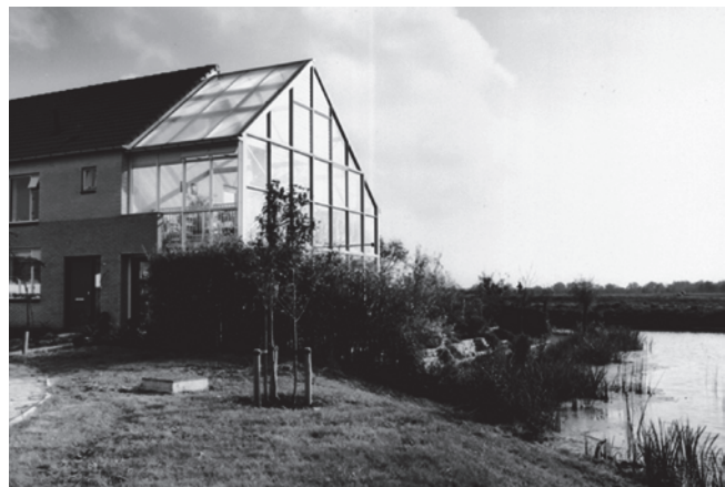
Fig. 05.37: Completed glasshouse dwellings in the Morra Park along the water front.
