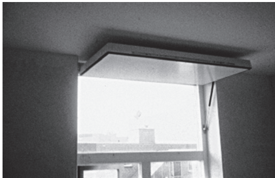
Fig. 05.31: Insulating shutter on the inside with a telescopic operation system (left) and fixed external sunshading (right).
