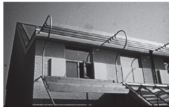
Fig. 05.31: Insulating shutter on the inside with a telescopic operation system (left) and fixed external sunshading (right).
