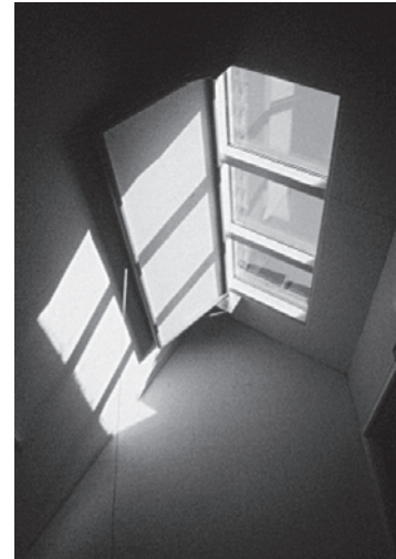
Fig. 05.14: Window (with shutter) in the upper roof on the south provides sunlight in the northern room.
