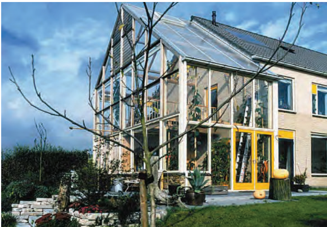
Fig. 05.33: Morra Park glasshouse; roofing of the glasshouse consisting of transparent three-layered corrugated plastic sheets.
