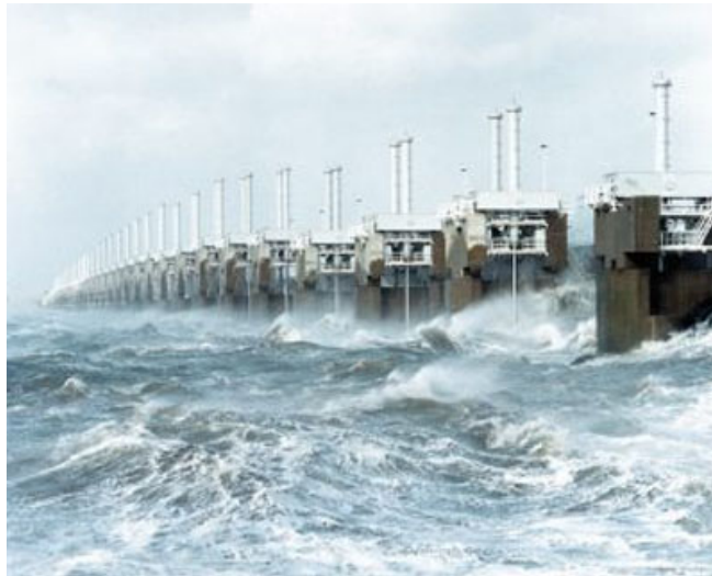
Figure A- 8 The Easter Scheldt storm surge barrier, The Netherlands [Source: Rijkswaterstaat].
