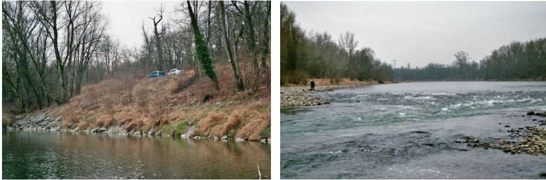
Figure A- 4 On the left the level difference is visible between the original river banks (where the cars are parked) and the current river bank. On the right the exposed rock on the river bed is shown in the upper Rhine at the border between Germany (left) and France (Right) [Source: E. Mosselman]
