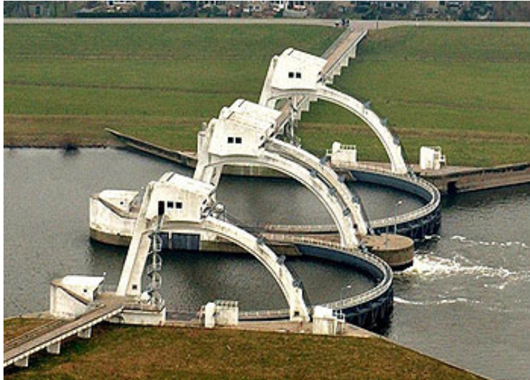
Figure A- 6 Movable Weir at Driel, The Netherlands [Source: www.driel.info ]
