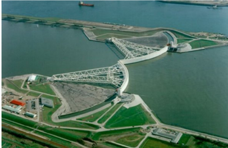
Figure A- 9 The Maeslant barrier, final piece of the Delta Works [Source: Van Wijngaarden Marine Services B.V.].
