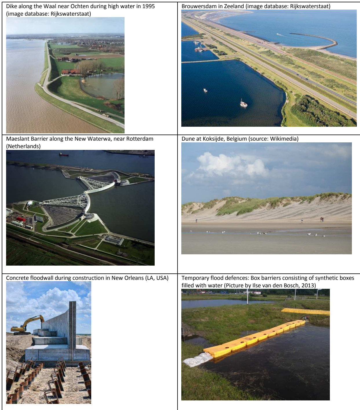
Figure 1: Overview of different types of flood defences
