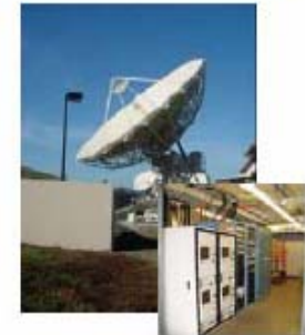
4 Ground Earth Stations
