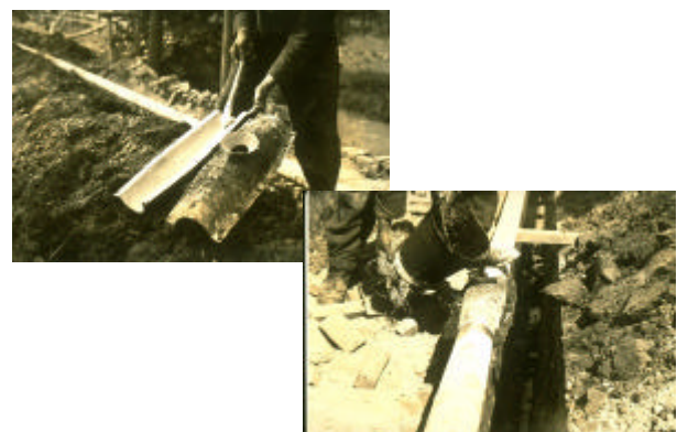
Fig. 2 - Hemp-lead joining of cast iron pipes
