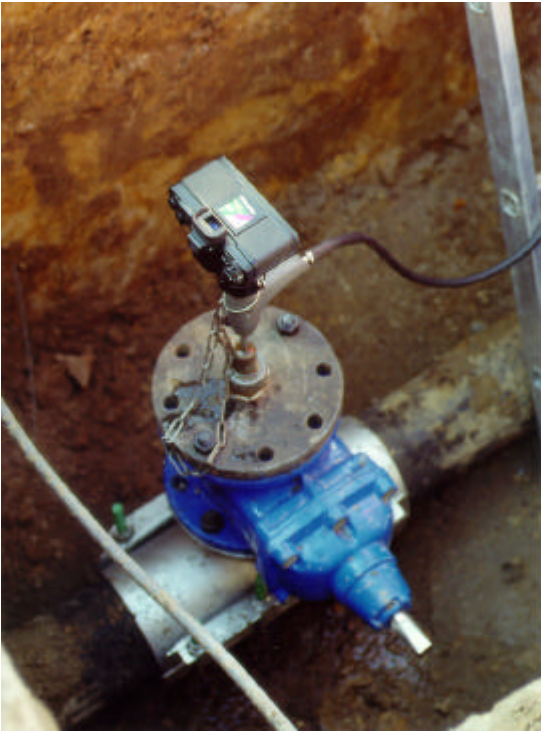
Fig. 9 - Camera for inspection of the pipe
