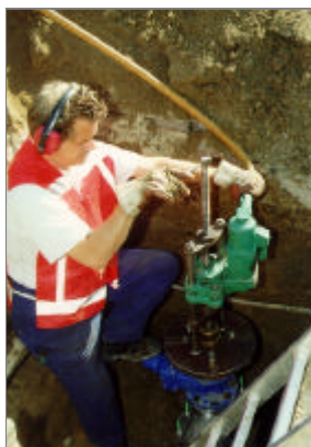
Fig. 6 - Coupon sampling
