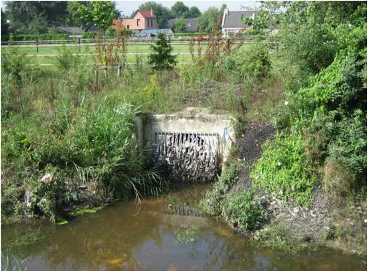
**Figure 4.8:** Outflow pipe of sewer overflow structure (weir is inside a manhole located at some distance inside the sewer system). The grid is applied to prevent playing children from entering the sewer system; the polluted fence leads to severe obstruction of the sewer outflow, which is likely to influence the overflow weir further upstream.
