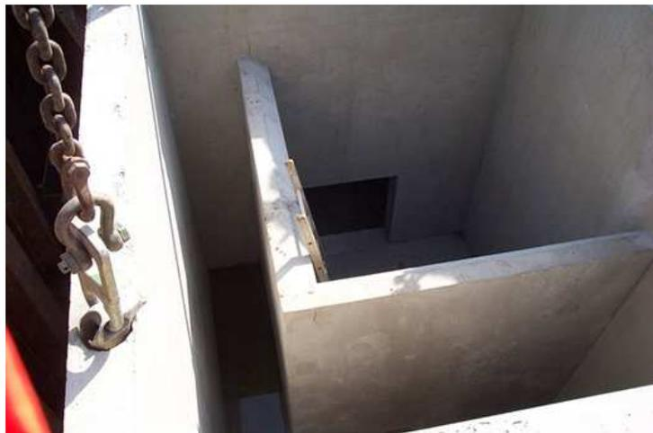
**Figure 4.7:** Overflow weir in sewer manhole during construction (Courtesy of Nederbetuwe)
