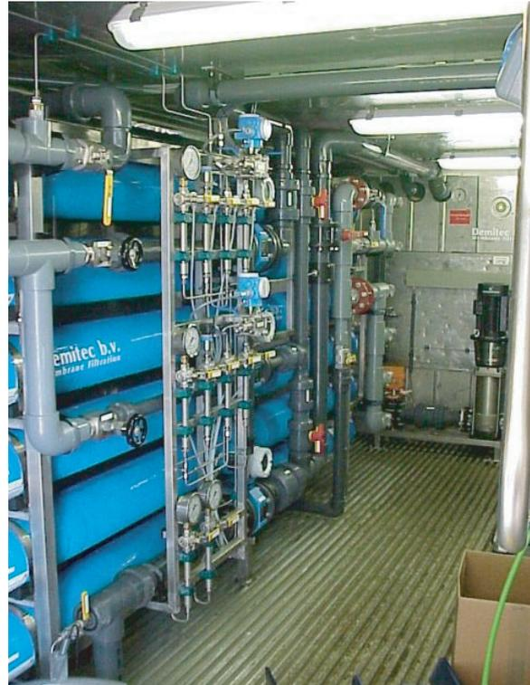
Figure 15 - Anaerobic NF-installation
