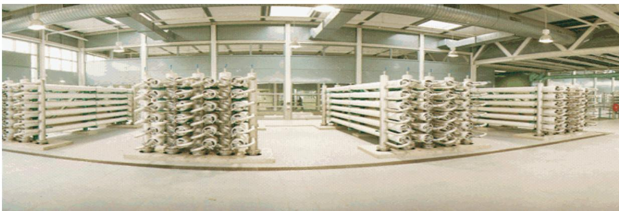
Figure 14 - Membrane installation at Heemskerk
