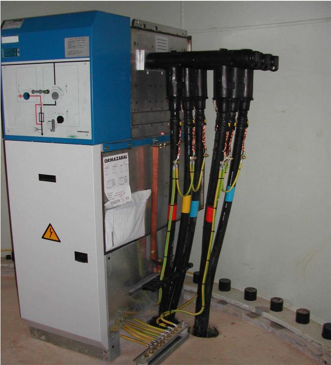
Figure 5. Ring Main unit arrangement
