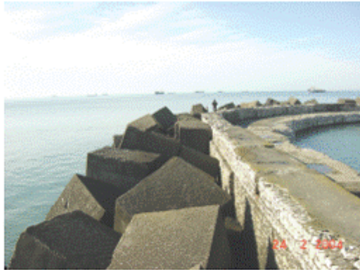
Figure 4 Breakwater chainage 0-1040 m
