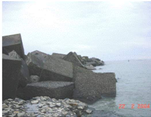
Figure 8 Breakwater chainage 1270-1810 m
