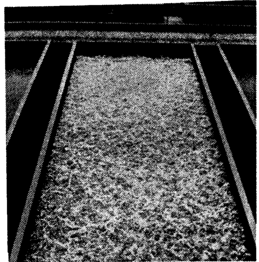
Fig. 3.31 Air wash prior to water wash
