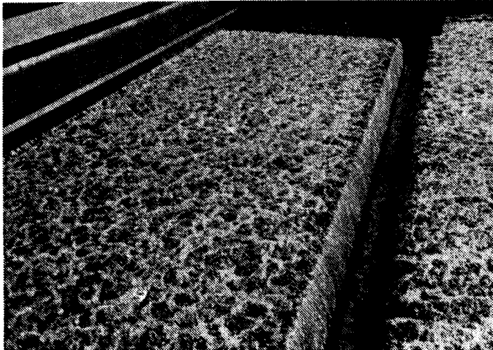
Fig. 3.32 Air wash combined with water wash
