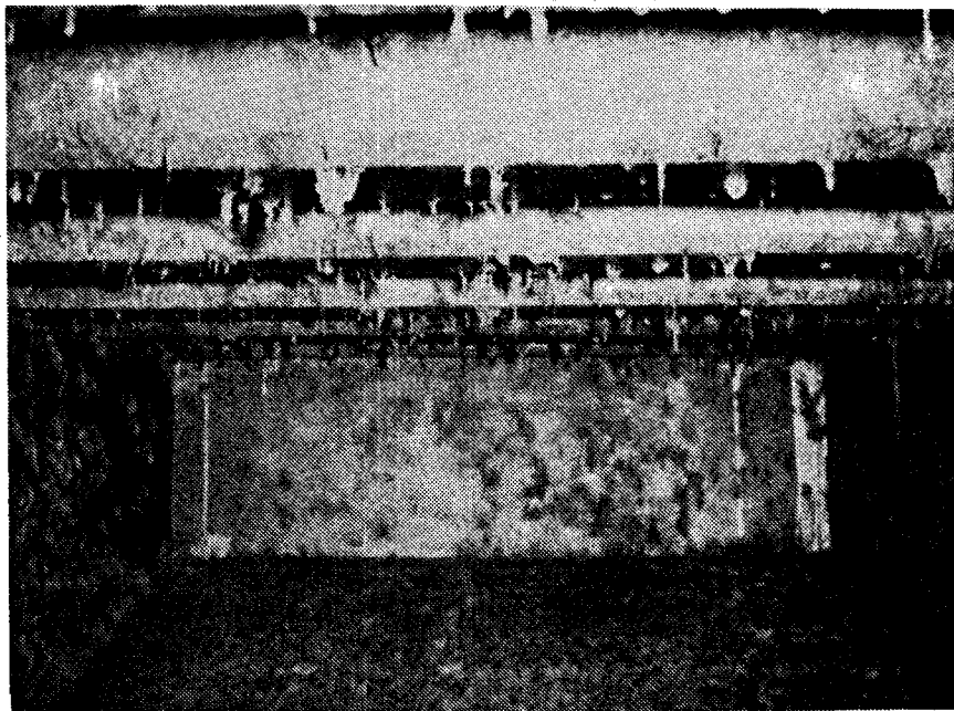
Fig. 4.33 Fouling of the space below a false bottom by aquatic growth
