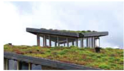
Fig. 2.9: Example of an extensive green roof
