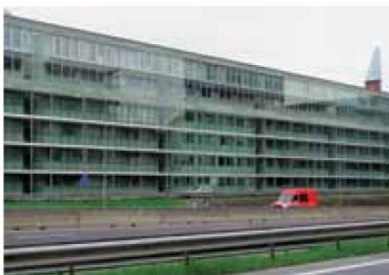
Fig 1.9: Renovation and construction project 'De Leeuw van Vlaanderen' with 72 rented apartments with a new double-façade as a noise barrier. To buffer noise and pollution from traffic on the A10 (Amsterdam) the second skin is placed in front of the existing east façade. The space behind this curtain wall serves to access dwellings and is ventilated with clean air from the west façade. Because of fire safety the glazed area is supplied with thrust ventilation to spread and disperse the smoke in case of fire.
