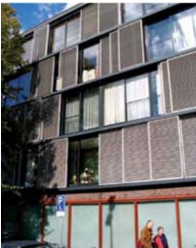
Fig. 1.5: Louver shutters or sliding screens: one of the many options for sun protection. The lamellae can be both fixed or rotated, depending on the type and make. The photo shows the project 'Delfts Blauw' with shutters made of an aluminium frame and lamellae. Producers are Limelight, developer and architectural firm Eurowoningen and Architecten Cie.
