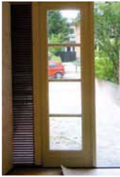
Fig. 3.11: Example of provision for a summer night cooling in a home in Zeist. The façade of the living room has two break free outlets ( 2 \times 2 \times 0.25 \text{ m} = 1 \text{ m}^2 ) with an insulated hatch. A skylight provides good natural draft. Ii architect studio realisation Ettehoven Contractor & interior decorator, consulting BOOM-SI, built in: 2009
