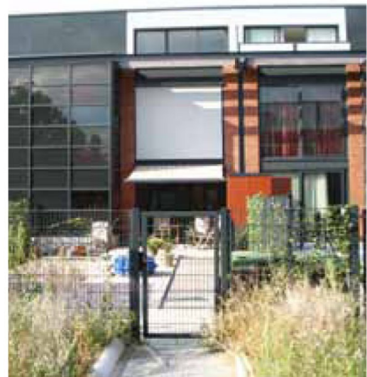
Fig. 2.29: Example of a project in which the movable blinds were included in the price. Part of the façade has transparent PV panels, also a form of sun protection. The dwellings are located in the energy district in Roomburg in Leiden
