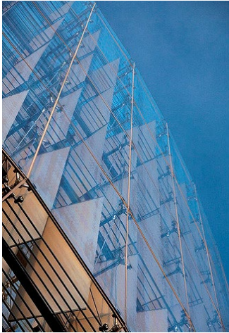
Fig. 1.14: double skin façade with shading applied in the cavity. Vivian and Seymour Milstein Family Heart Center, Photo credit: Paul Warchol
