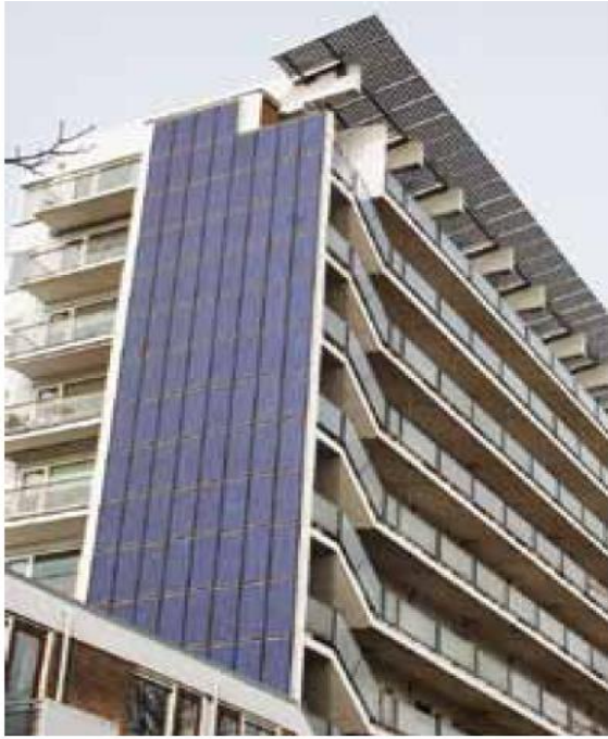
Fig. 1.6: In the sustainable skyscraper redevelopment Bieslandsekade by Woonbron Delft, a total of 260 m 2 PV panels were installed during the refurbishment. The PV panels are integrated into the façade, roof and balconies. The PV panels on the roof also serve as sunshades and those on the balconies at the same time ensure privacy. The solar electricity generated provides nearly all public facilities in the ten-story building such as lifts, lighting and mechanical ventilation. Client: Woonbron, Architect: Van Schagen architects, engineering and installation PV: BST, Elektron, advice: W / E consultants. Built in: 2003
