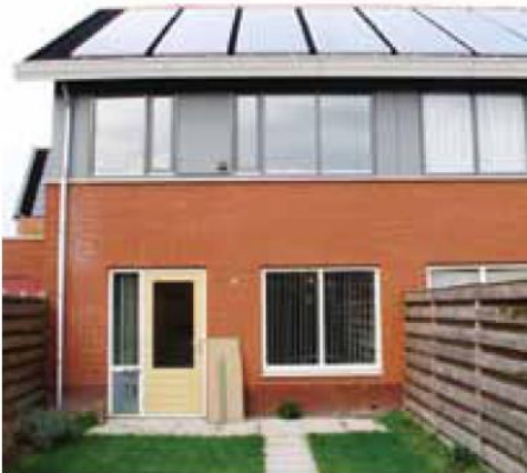
Figure 1.5 An example of integrated PV panels in a roof. This is the 'Stad van de zon' (city of sun) demonstration project. Each roof has 3600Wp installed. The yield is around 3400 kWh/yr. This type of PV was awarded the 'Dakaward' (roofaward) 2004. Design BBHD architects, Development VBM (vos Alkmaar) Projectleader Willem Koppen, contractor Heddes Bouw, PV producer BP-Solar, built in: 2003
