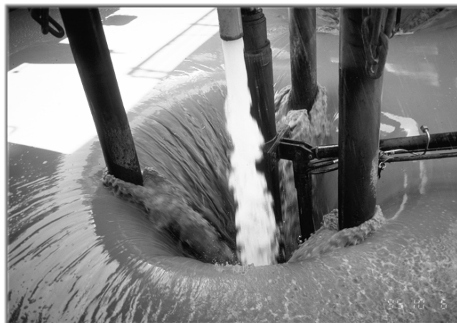
Figure 2-102 Standard adjustable overflow.
