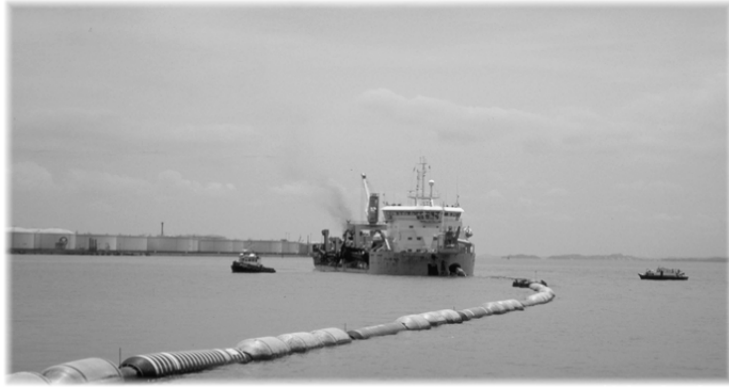
Figure 2-11 TSHD J.J.F. de NUL picking up the floating pipeline to the shore connection
