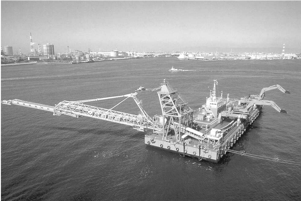
Figure 5-2 A Japanese BUD with backhoe's and belt conveyors.
