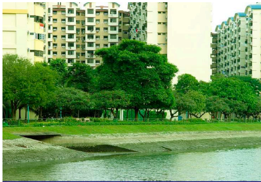
Kolam Ayer Project - Before
