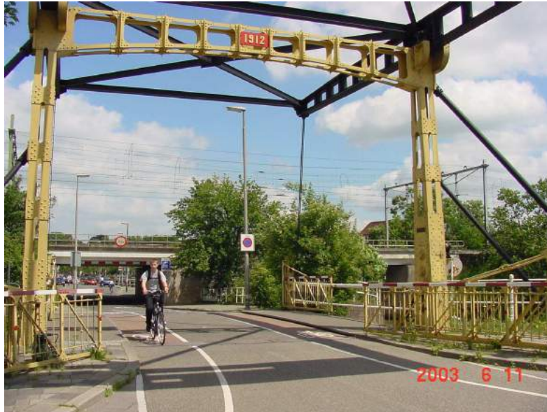
Fig. 516 Neighbourhood street crossing canal and railroad in Utrecht
