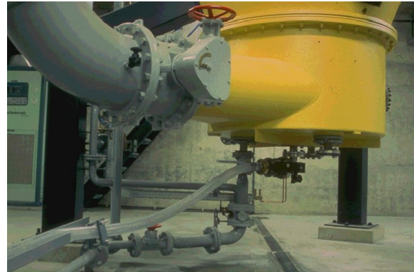
Figure 20 - Tangential flow of raw water
