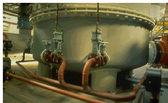
Figure 21 - Several pipes at the bottom of a pellet reactor
