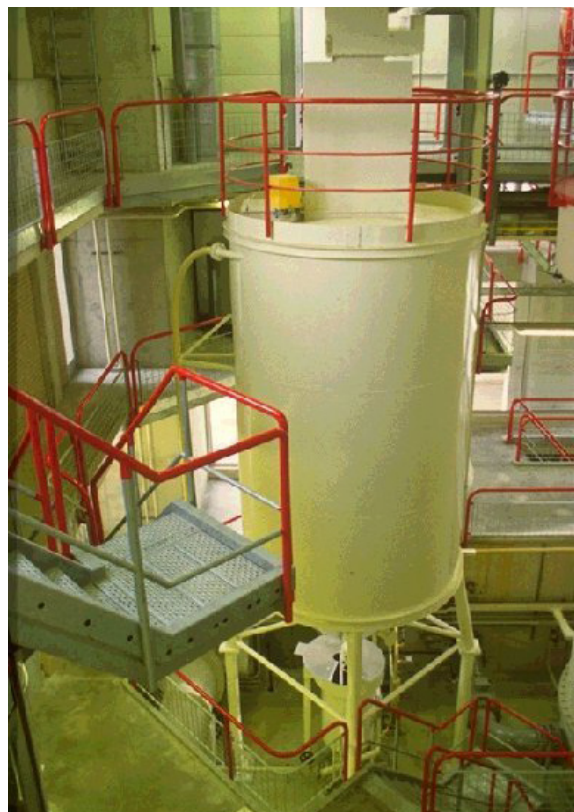
Figure 23 - Seeding sand storage silo with sand washer underneath
