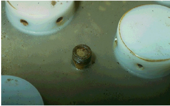
Figure 16 - Dosing system with separate caustic soda and water dosing nozzles in the bottom
