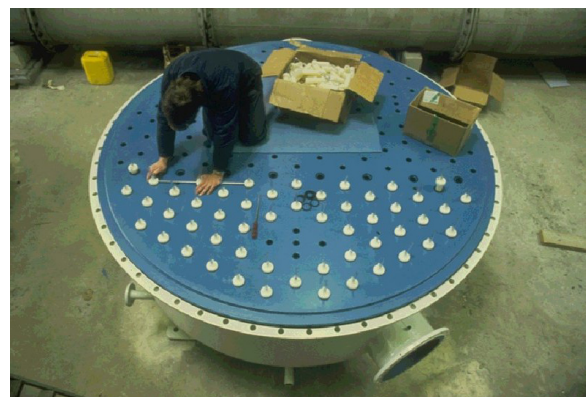
Figure 15 - Dosing system with separate caustic soda and water dosing nozzles in the bottom
