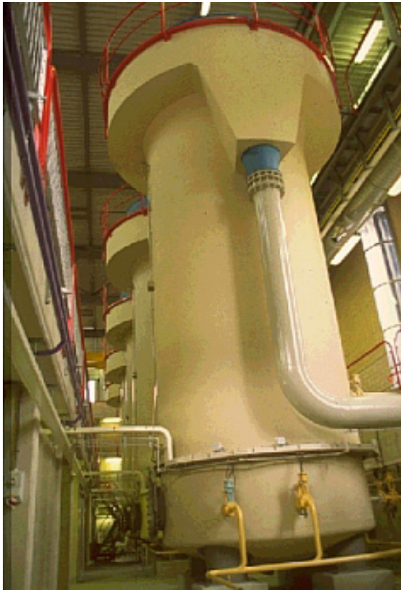
Figure 2 - Pellet reactor used for softening of drinking water
