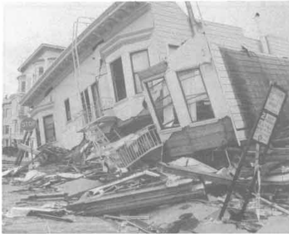
Figure 1-5a: Structural devastation causes loss of life and capital. This house in the Marina district, San Francisco, collapsed during the October 17, 1989, Loma Prieta earthquake.
