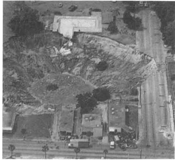
Figure 1-8a: Sinkhole of Winter Park, Florida, formed May 7, 1981.
