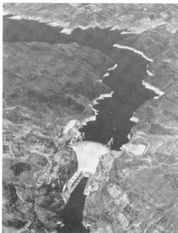
Figure 1-9c: Geological site investigations ensured the stability of the walls and floor of the Colorado River, supporting the Hoover Dam, Nevada.
