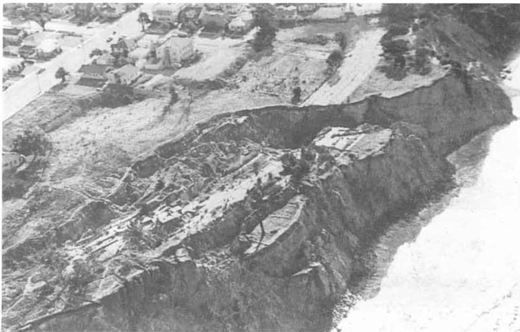
Figure 15-12: Collapse of urbanized cliffs at Point Fermin, California.
