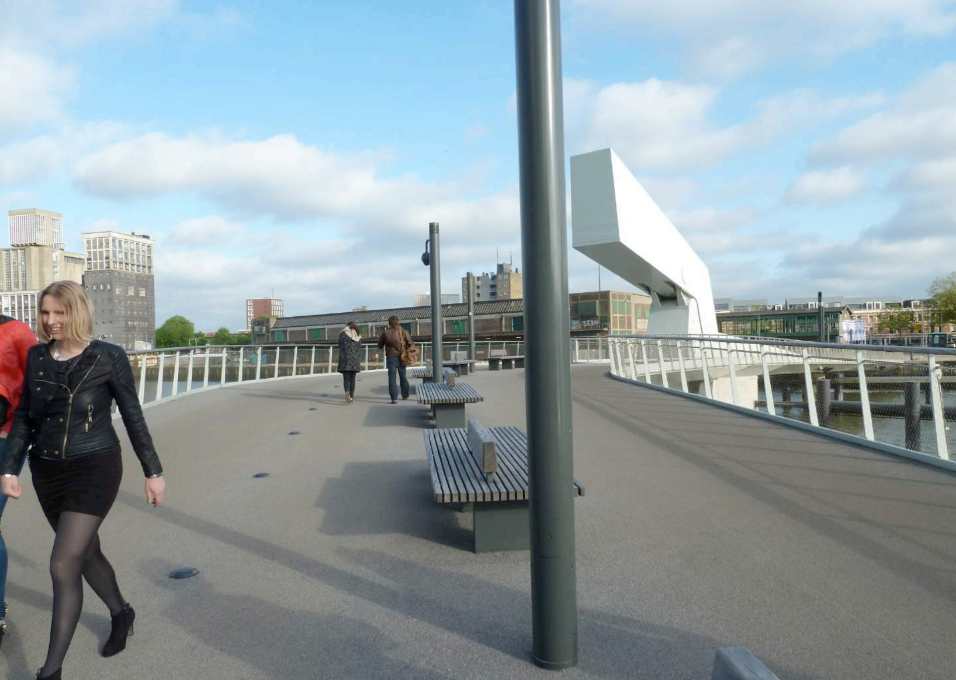
New pedestrian bridge between Wilhelminapier and Katendrecht
