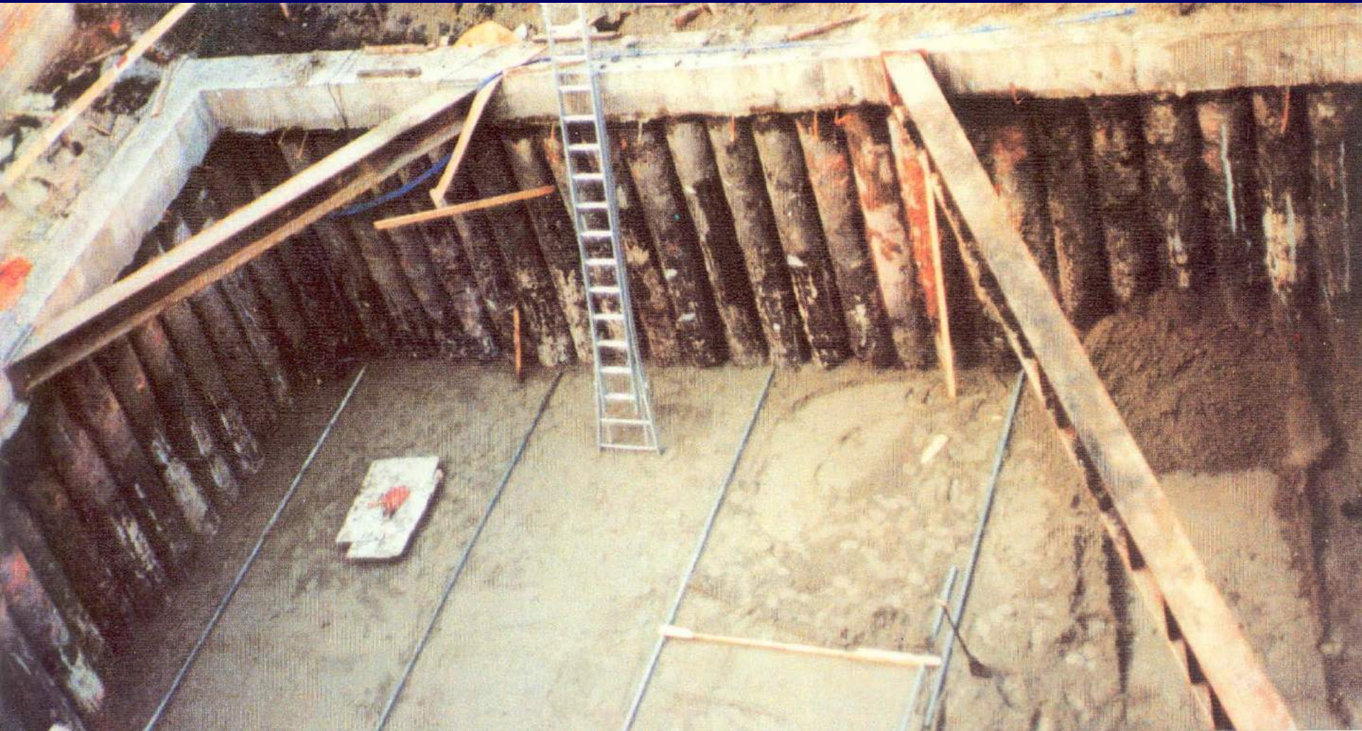
Building pit with auger pile wall
