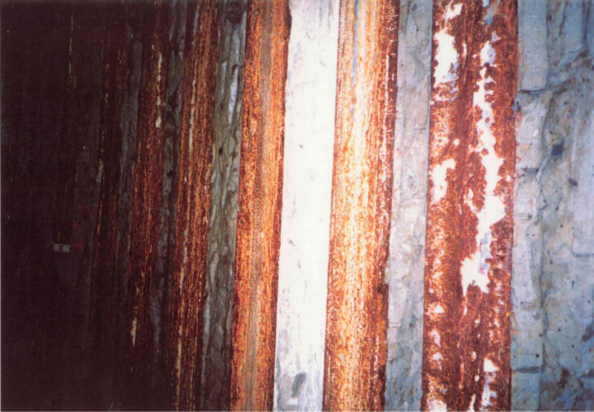
Mixed in place, strengthened by steel profiles
