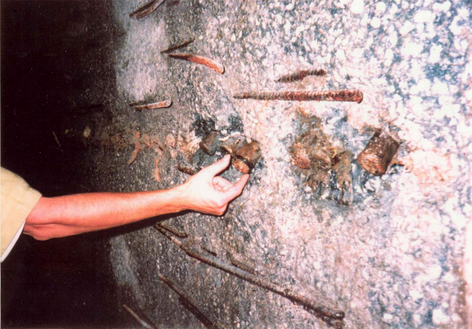
Diaphragm wall at 25 meter minus (connection screw housing and starter bars)
