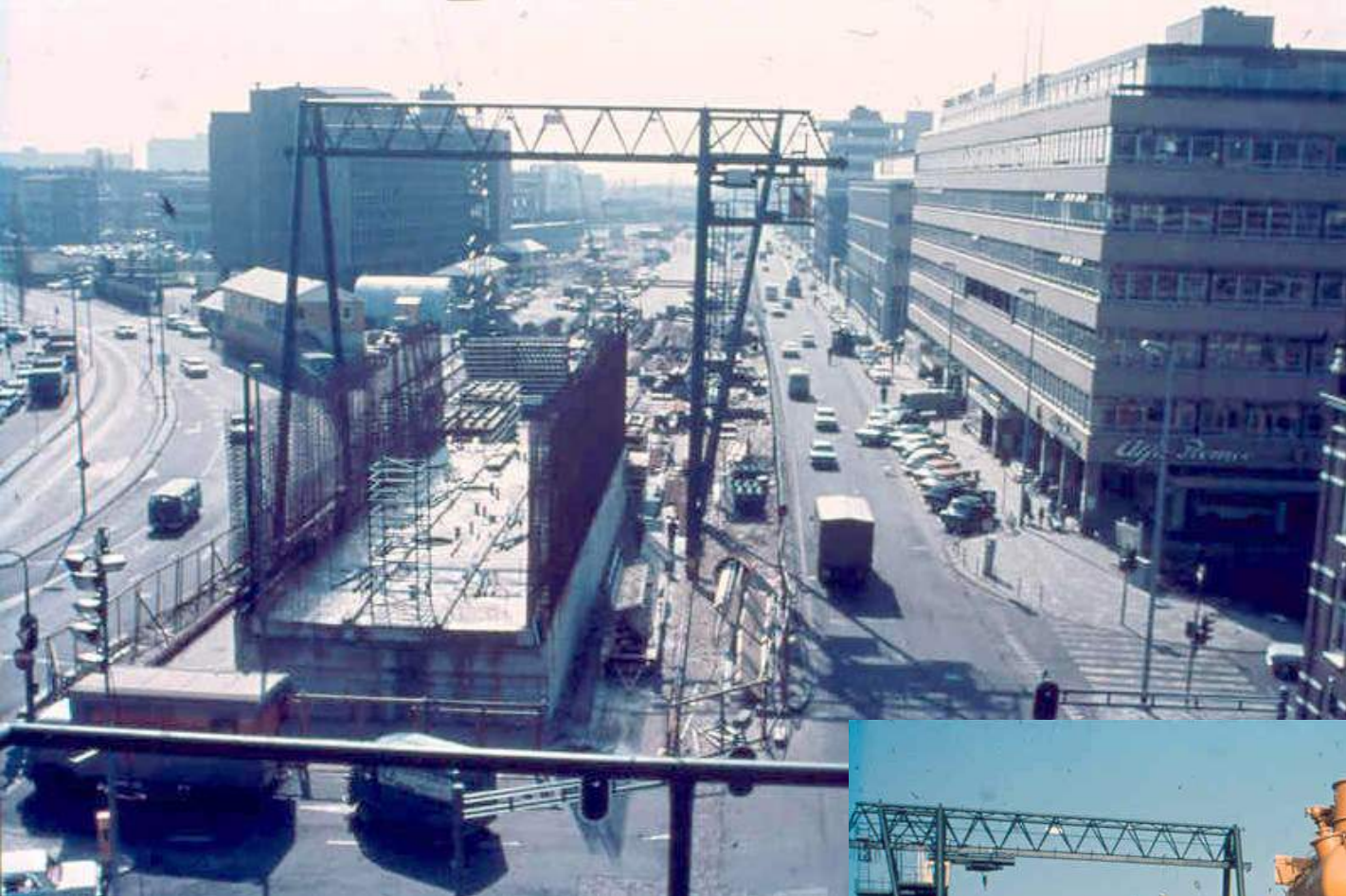
Construction of a caisson
