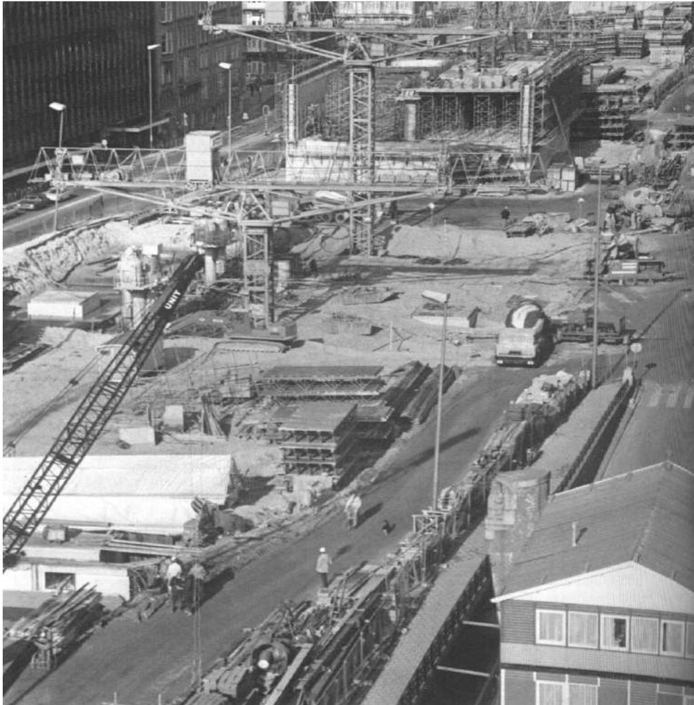
Figure 7.4: Caissons for the East-line of the Amsterdam subway under construction
