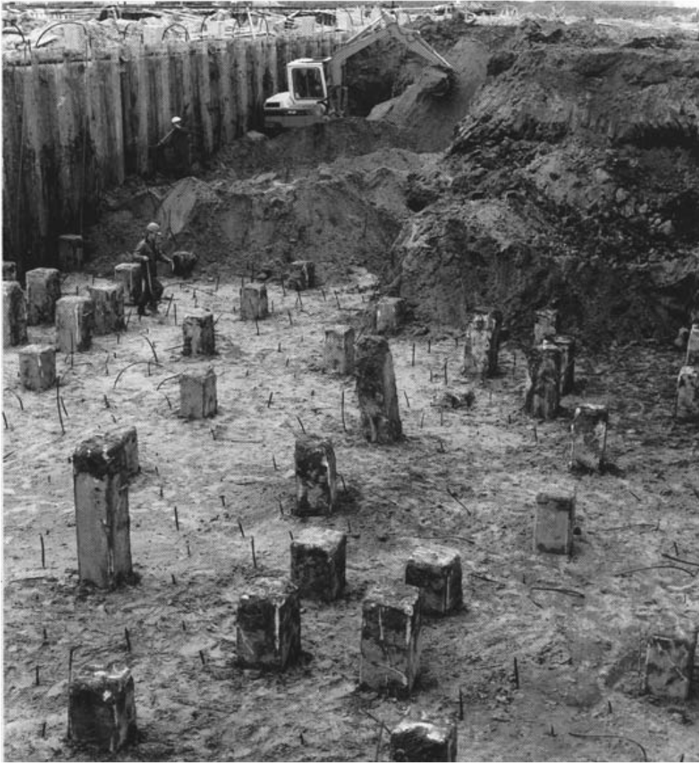
Figure 3.6: Example of soil injection for soil improvement.
