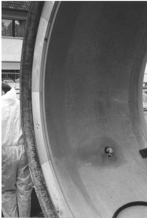
Figure 11.14 Bore pipe with bentonite – injection points
