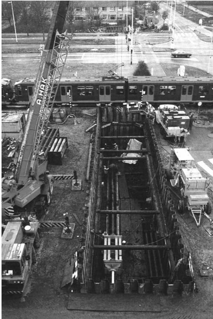
Figure 11.15: Jacking shaft for drilling under railway
