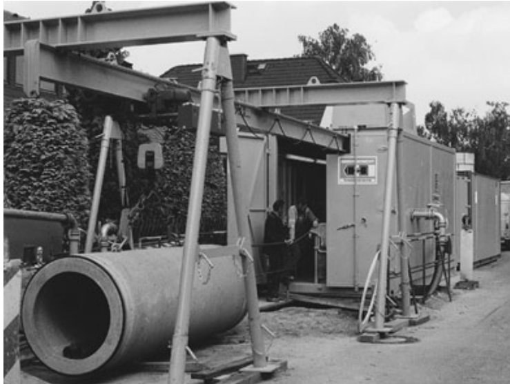
Figure 11.10: Hoisting of a concrete pipe
