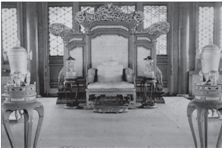
417 Stage IV Study of material and construction
