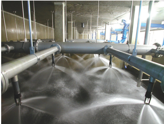
Figure 12 - Aeration over a dry filter in Zwijndrecht (Zuid-Holland)
