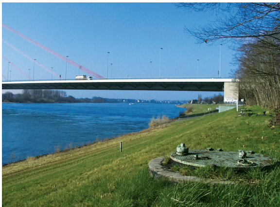
Figure 10 - Riverbank groundwater well in Germany
