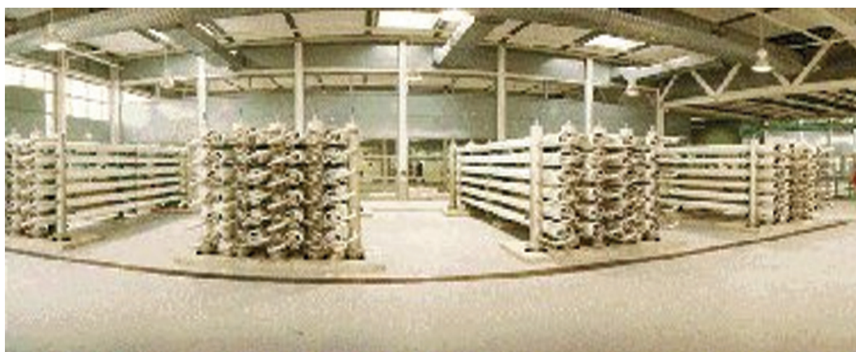
Figure 23 - Membrane filtration plant in Heemskereek (Noord-Holland)
