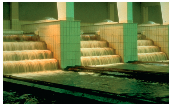
Figure 7 - Treatment of slightly anaerobic groundwater
