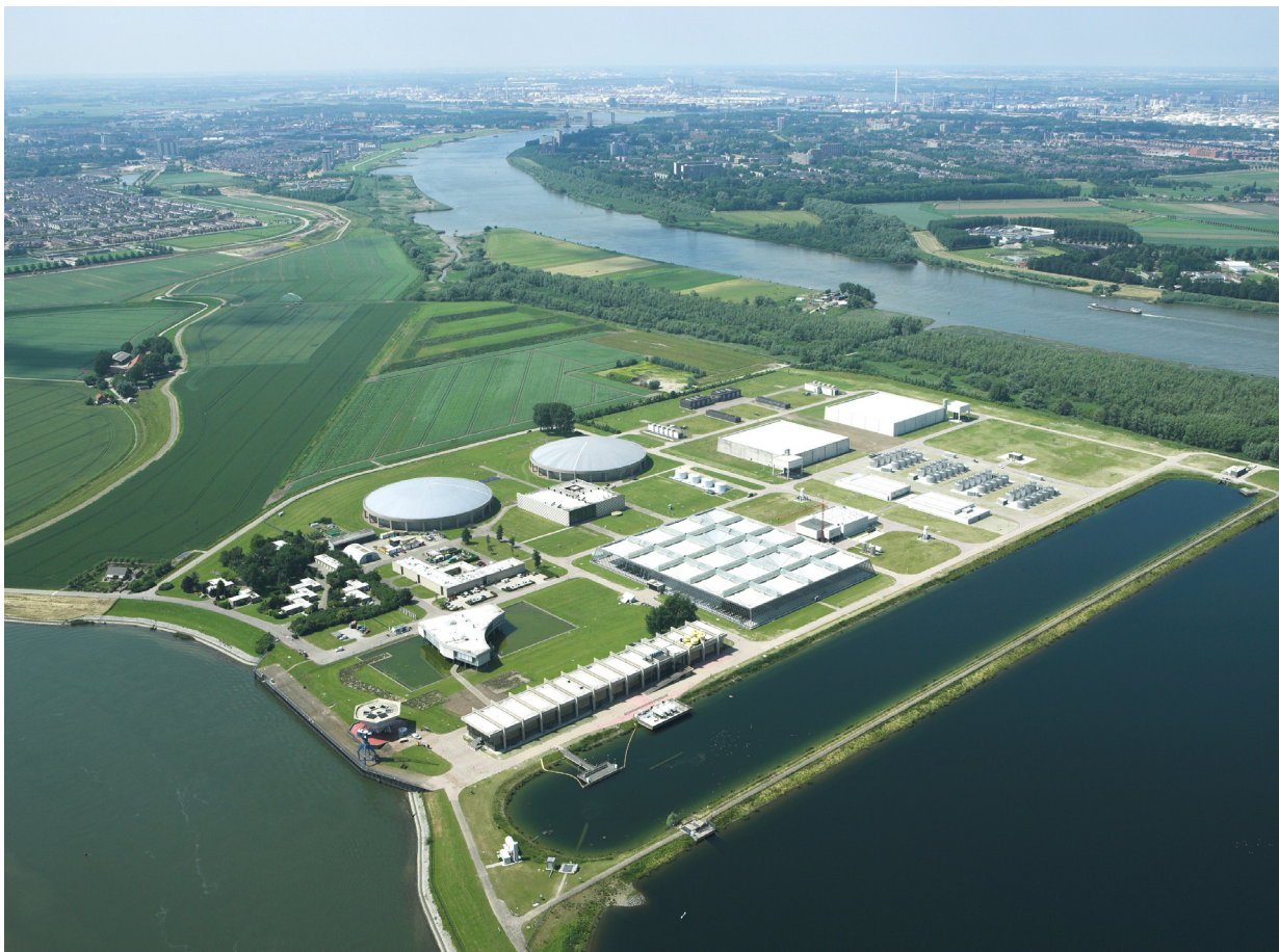
Figure 15 - Drinking water production at the Berenplaat production plant (Zuid-Holland)
