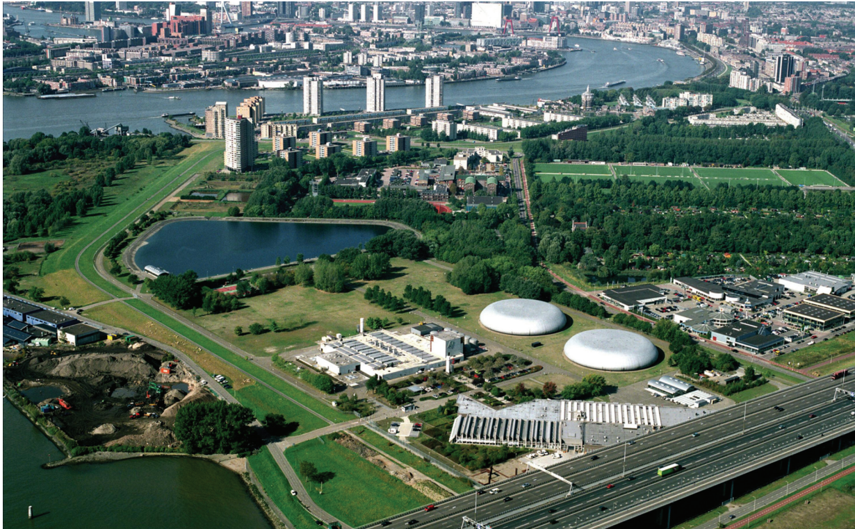
Figure 17 - Kralingen drinking water production plant
