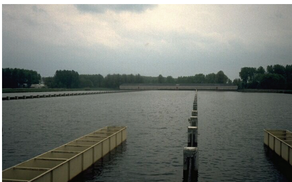
Figure 28 - Open sedimentation pond at Nieuwegein (Utrecht)
