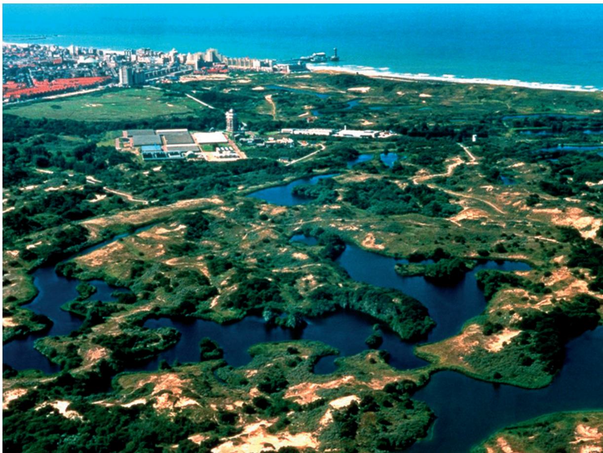
Figure 31 - Infiltration area and post-treatment plant near Scheveningen
