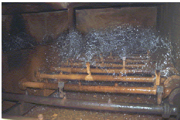
Figure 4 - Aeration above limestone filter
