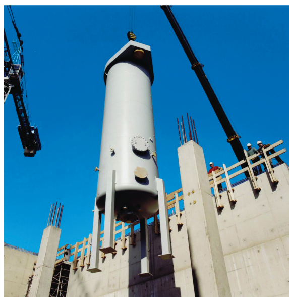
Figure 5 - Pellet reactor for softening water in Meerssen (Limburg)
