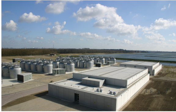
Figure 19 - UV disinfection (right) followed by activated carbon filtration (left) at Berenplaat production plant (Zuid-Holland)
