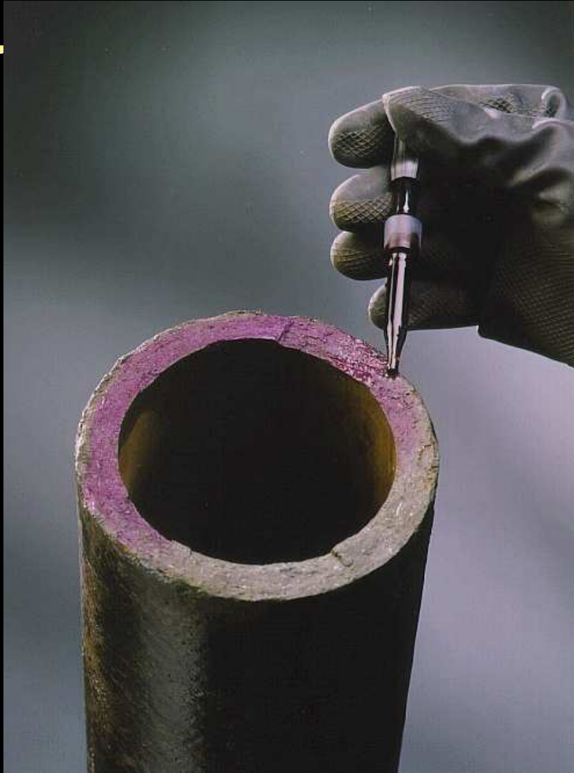
Operation and maintenance of networks
