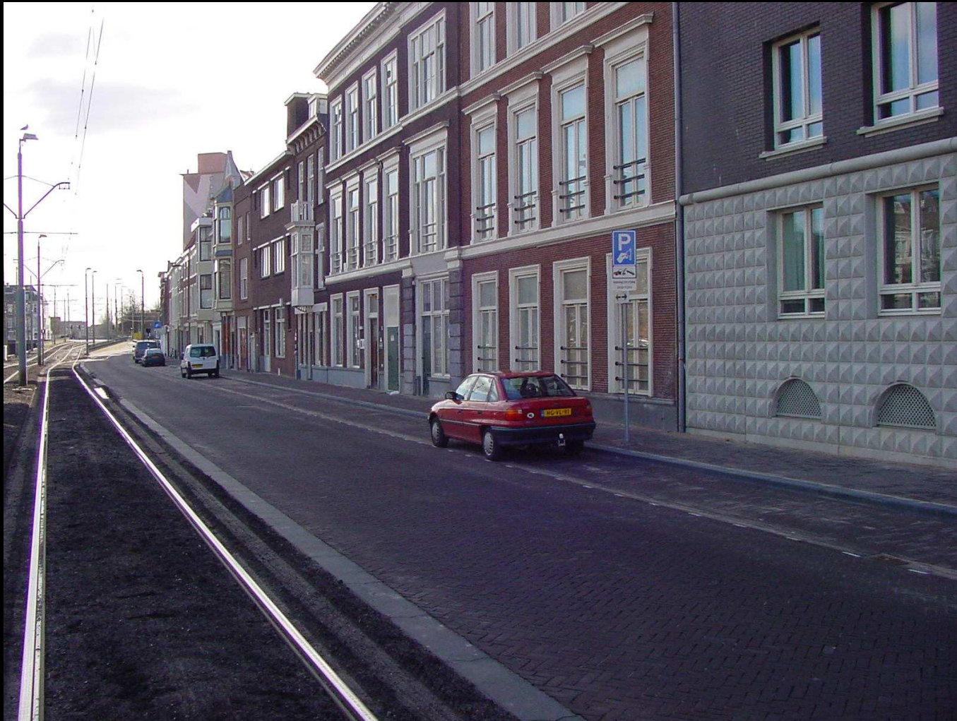
Operation and maintenance of networks
