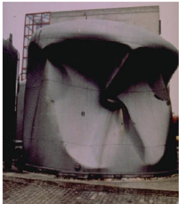
Fig. 2.16 - Imploded tank
