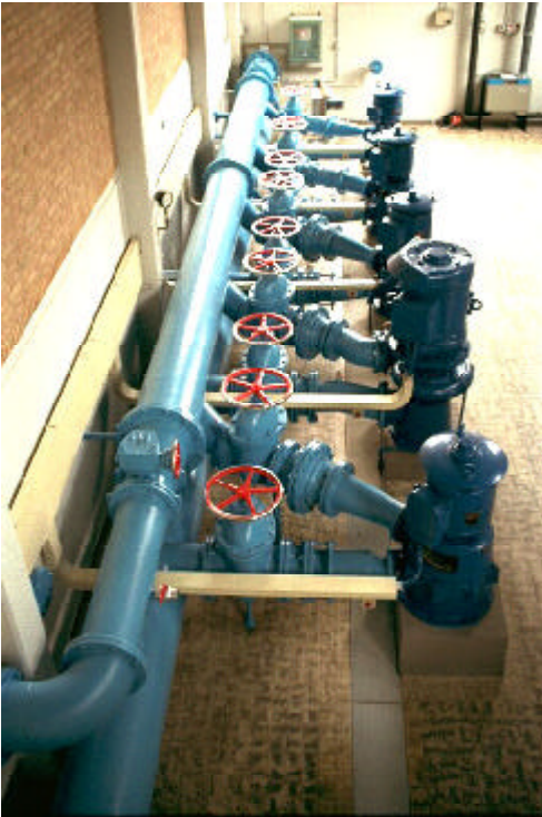
Fig. 3.23 - Multiple pumps in parallel
