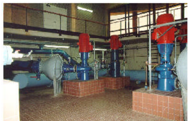
Fig. 3.29 - Pump with non-return valve
