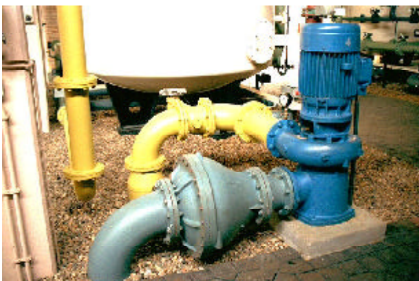
Fig. 3.31 - Pump with check valve
