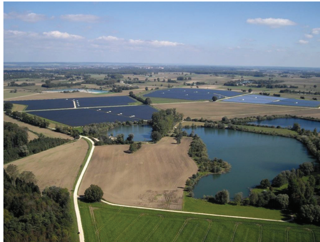
Figure 17.4: The 25.7 MW p Lauingen Energy Park in Bavarian Swabia, Germany [136].
