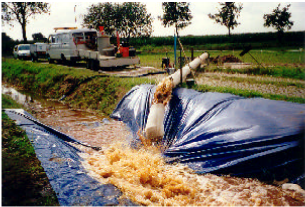
Fig. 7.12 - Foam pig leaving a pipe
